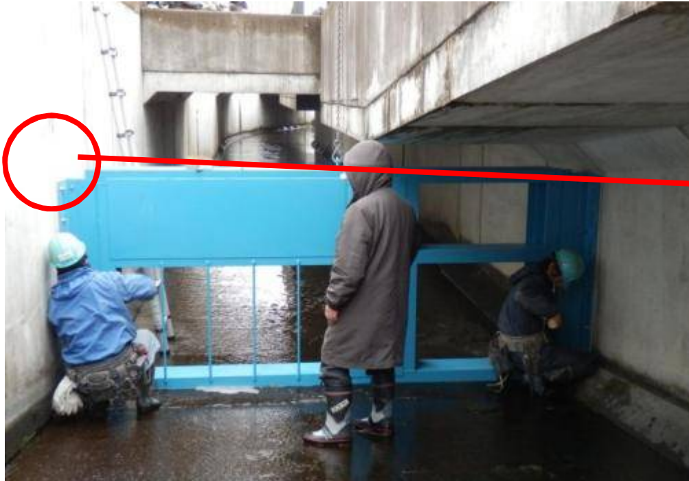
Setting the control gate and prevention of leakage
