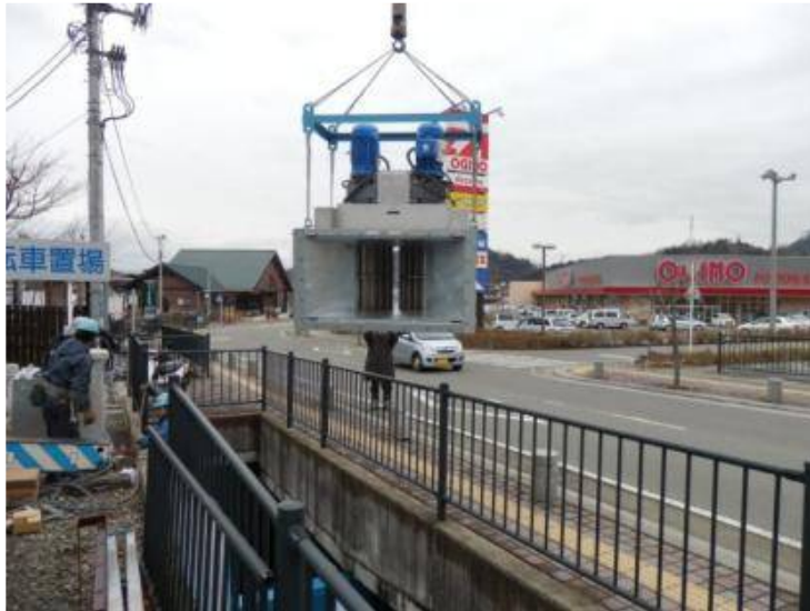
Lifting to install the system
