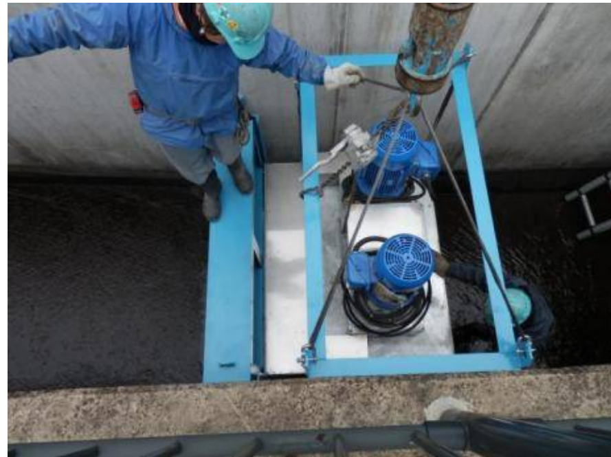
Adjust by horizontality, height, and direction.
