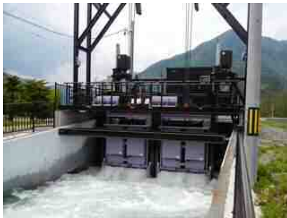
A Irrigation canal, Nagano pref. / rated output : 37kW x 2units / Mar. 2017
